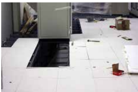
Supporting floor tiles
